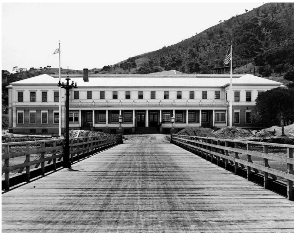
Wharf and administration building, Angel Island Immigration Station, c. 1910. Despite strident protests by the Chinese American community, the immigration station on Angel Island was opened in January 1910. The station was considered “ideal” because its island location made it escape-proof. Courtesy of the National Archives, Washington, D.C.
